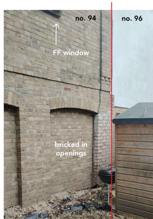
Existing Rear Elevation View from 94 Cliff Road rear garden
