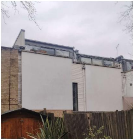
Rear windows to no.96 - 100
