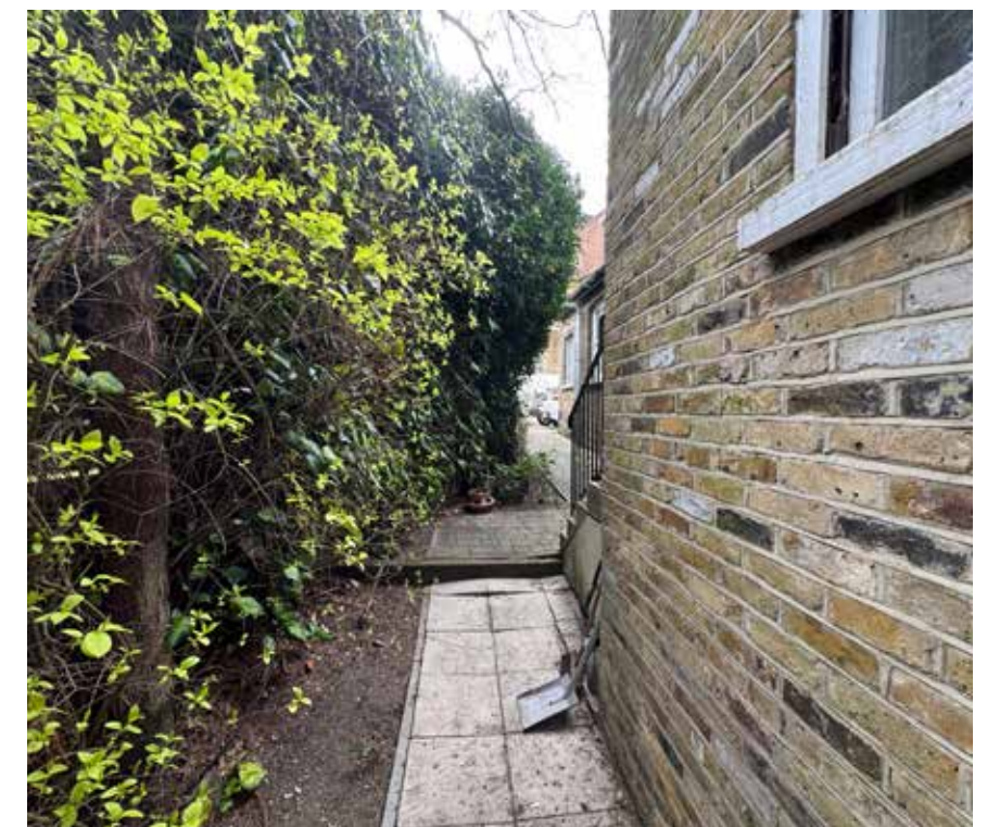
Fig.30- Narrow and uneven perimeter path from ramp
