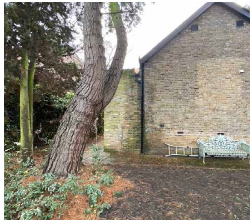
Fig.22- T2 Tree in foreground, blank north elevation of existing house
