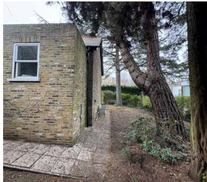
Fig.29- No access to garden from rear of property
