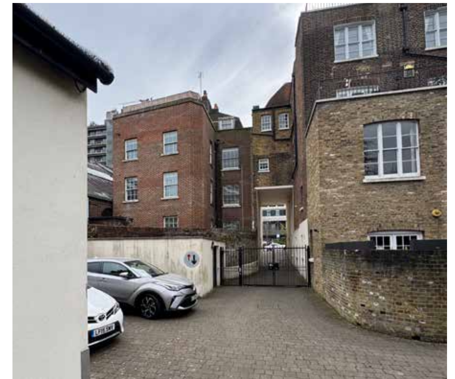
Fig.23- 21 + 23 Pond Street overlooking Pond Court and Connaught Mews
