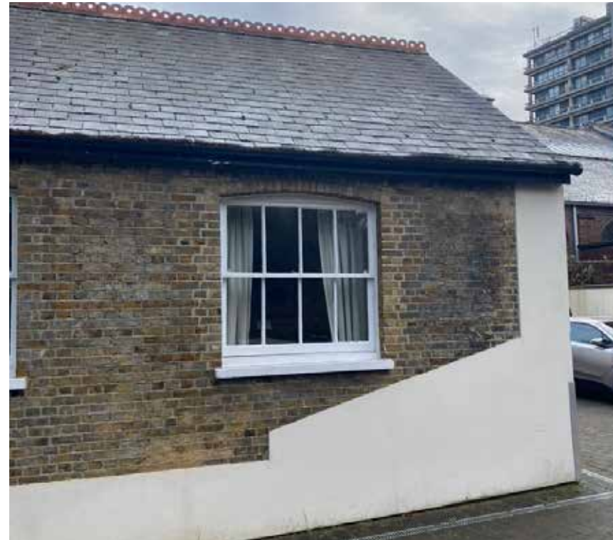
Fig.14- West Elevation- london stock brick,/ partial render, segmental arches, timber sash windows
