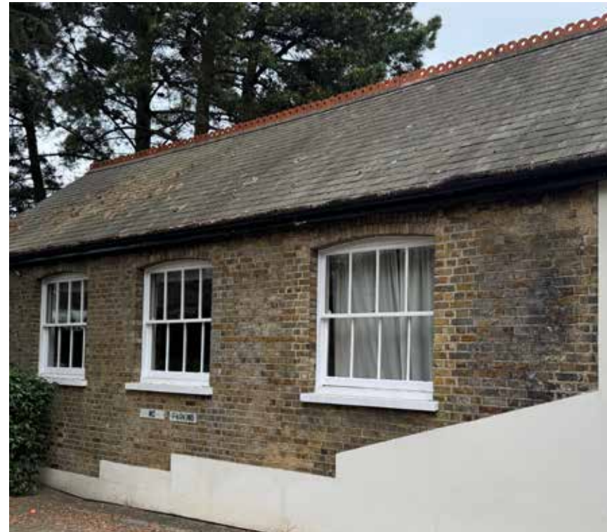
Fig.53- Existing slates to be replaced with new natural slates to match existing
