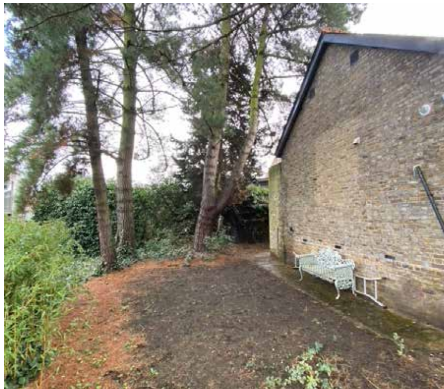
Fig.16- North Elevation currently without fenestration and in solid brickwork
