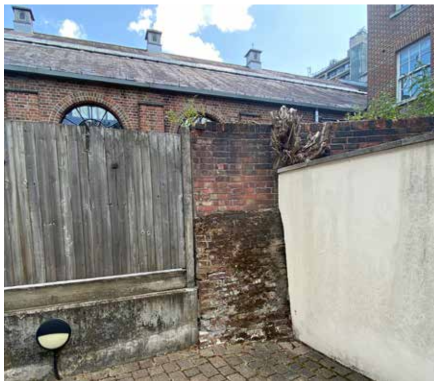
Fig.24- Boundary wall from 23 Pond Street terminates adjacent concrete wall and fence over
