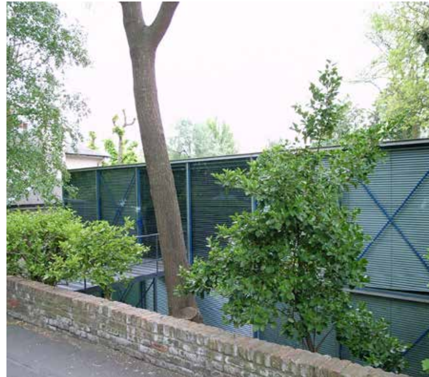
Fig.37- 49a Downshire Hill NW3 Completed 1978
