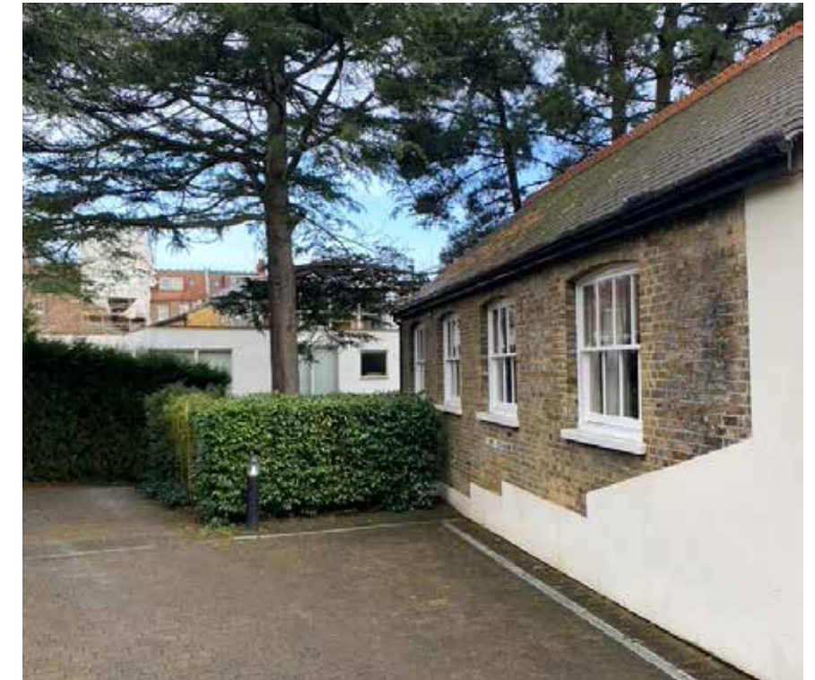
Fig.15- West Elevation looking north to Monterey Pine Trees
