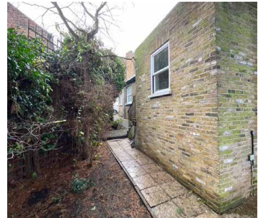
Fig.18- Later flat-roofed side addition. Later sash window with shallow reveal and flat brick arch
