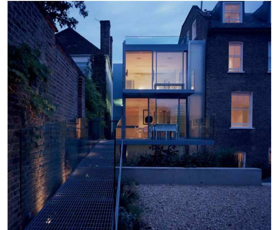
Fig.38- Pilgrims Lane by Eldridge Smerin Architects- completed 2010
