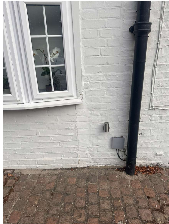
B. Existing front elevation – showing poorly detailed and fitted UPVC window fenestrations
