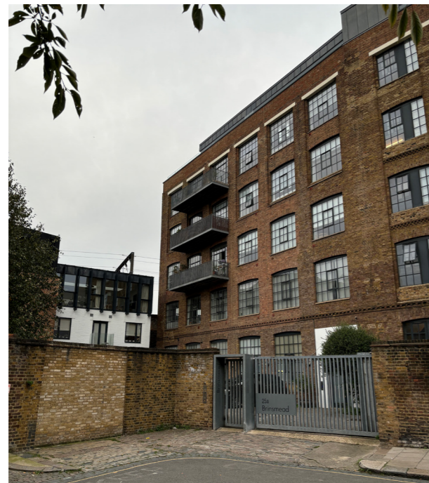
View of 25a Ryland Road - Brinsmead Apartments
