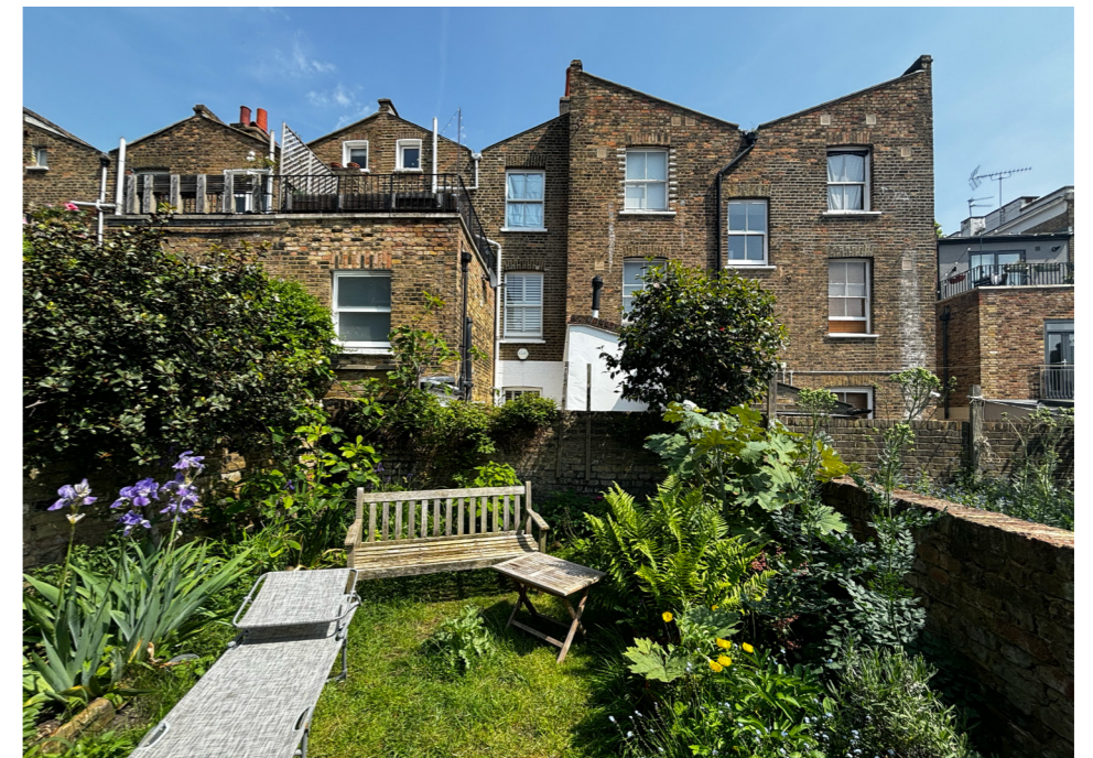
View from garden of 15 Ryland Road onto rear facades of Grafton Road
