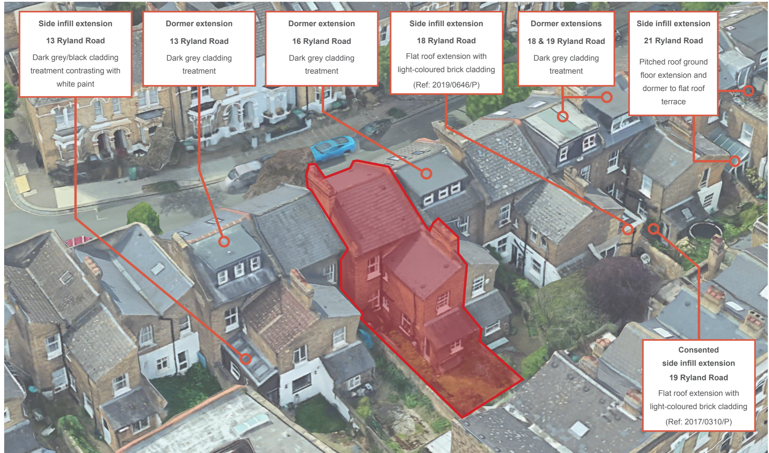
Aerial view of 15 Ryland Road from the south-east showing the ad-hoc nature of the existing terrace row
