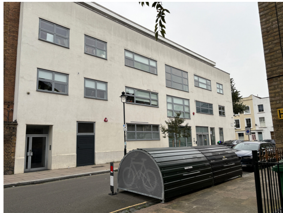
View of 24b Ryland Road
