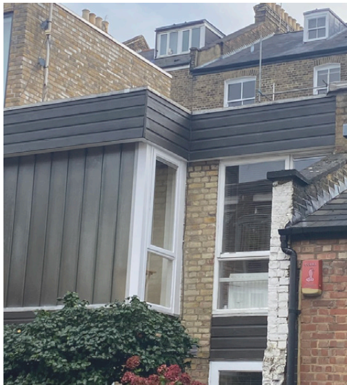
Facade of brick, channel glazing, and timber
