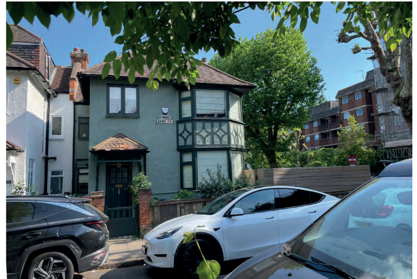
No. 23 Glenhurst Avenue - north elevation from Glenhurst Avenue May 2026
