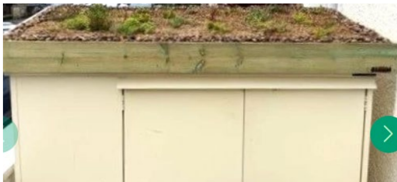
Figure 3: Example of green roof on Asgard Bike Shed on found elsewhere in London
