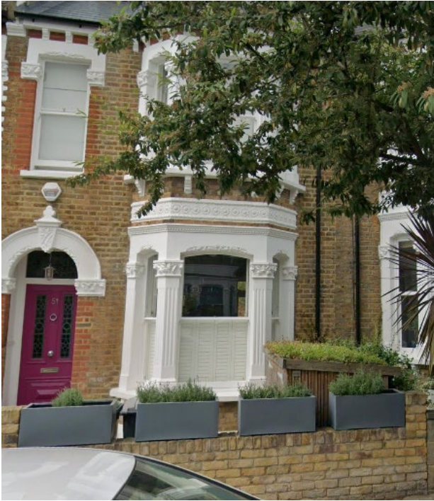
Figure B4: 51 Solent Road – Wooden Bike Shed, with green roof. Same Size and Scale as proposed application (Google Street View)
