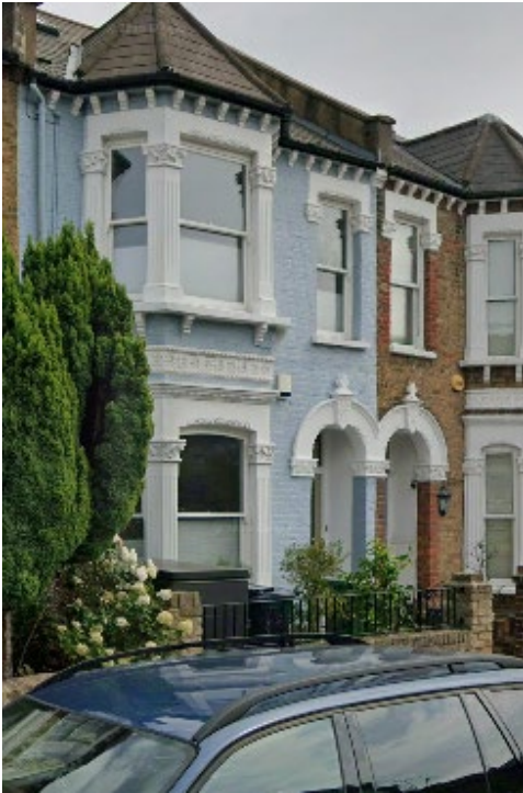
Figure B1: 4 Solent Road - metal Asgard-type bicycle storage unit visible in the front garden (Google Street View)
