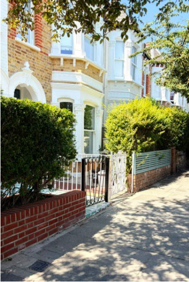
Figure 2: Current oblique view of the property showing no change to front view and with bike shed in situ
