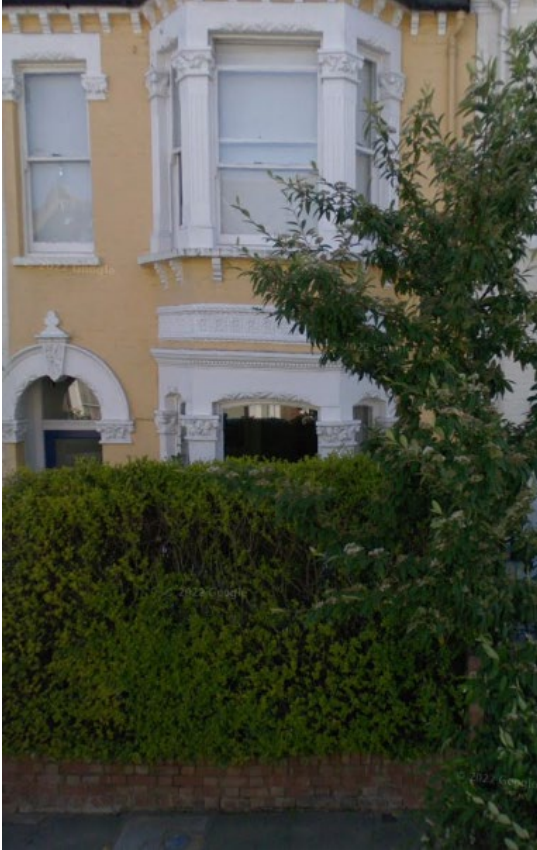
Figure A1: 29 Solent Road - front boundary hedge, Google Street View 2008, confirming the hedge was well-established over 17 years ago
