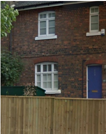
Figure H2: 210 Iverson Road, Approved Metal Unit
