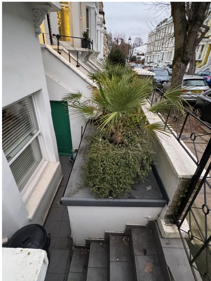
front facade sunken patio
