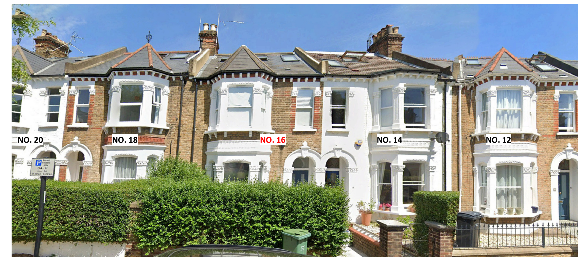
IMAGES OF EXISTING - SOUTH ELEVATION LOOKING AT 16 SOLENT RD WITH 14 & 12 SOLENT RD TO THE RIGHT AND 18 & 20 SOLENT RD TO THE LEFT.
