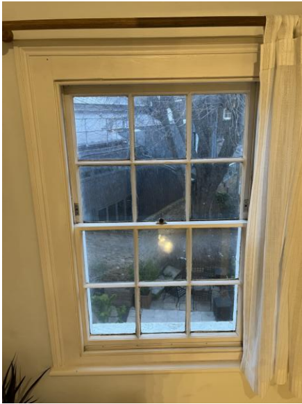
Stairs rear sash window
