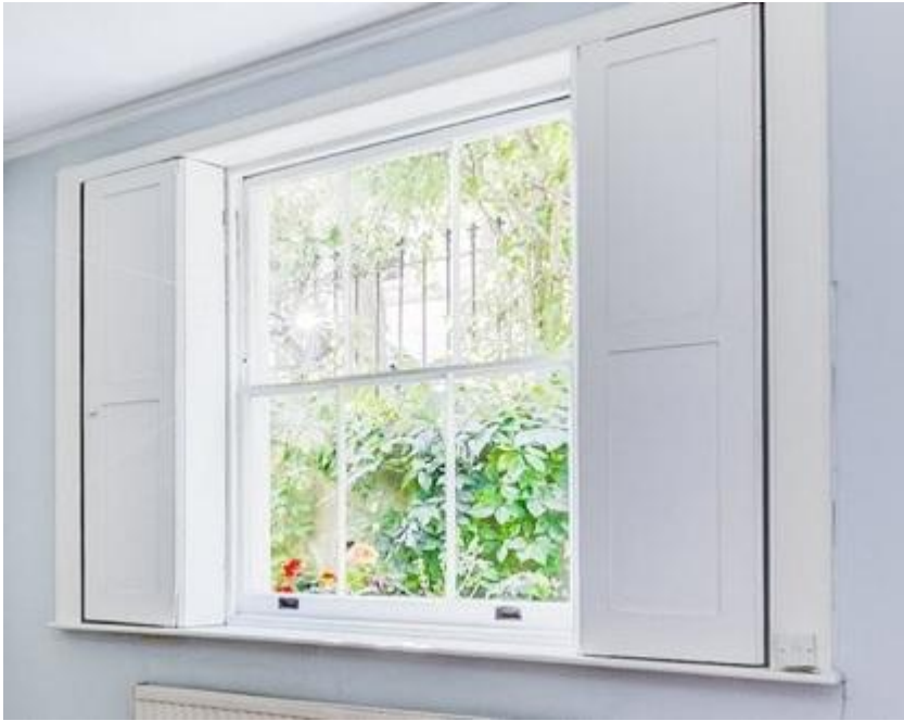
Lower ground front sash window
