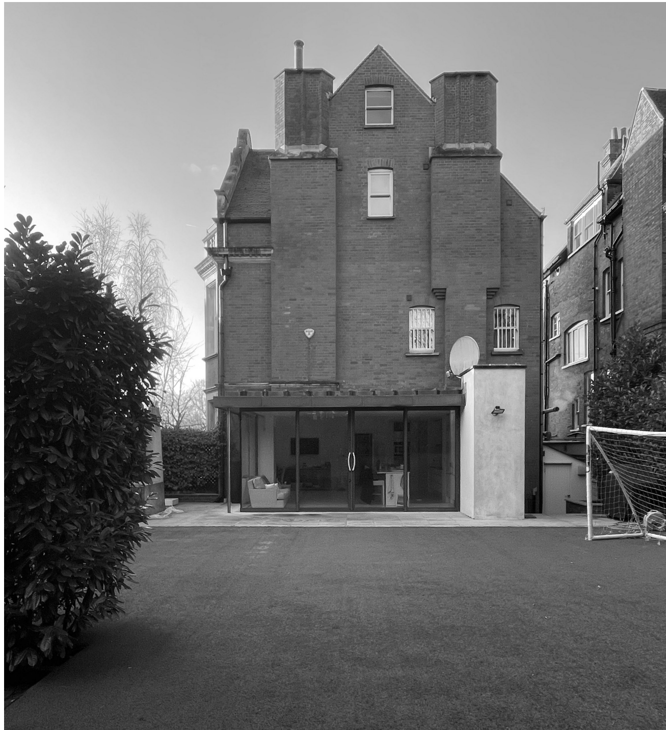
04. Existing Building - Current rear extension
