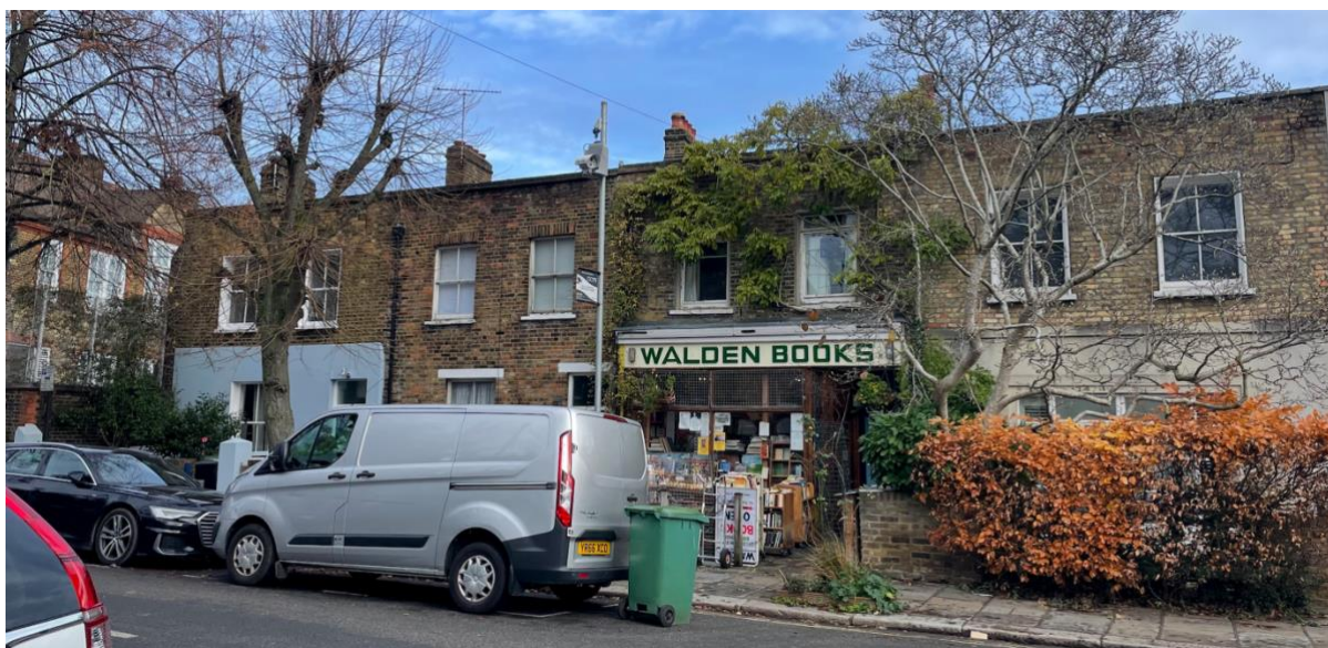
Figure 15: The terraced group that contains the subject site (far left) and the book shop (No. 38)
