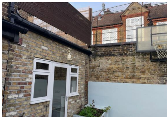
Figure 11: Looking northwards towards the boundary with the school with wire high level fencing over brick wall
