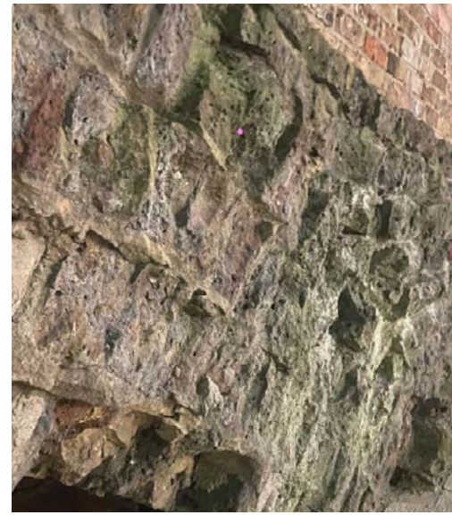
P2 - Remains of arches visible at lower ground floor level indicates vault presence
