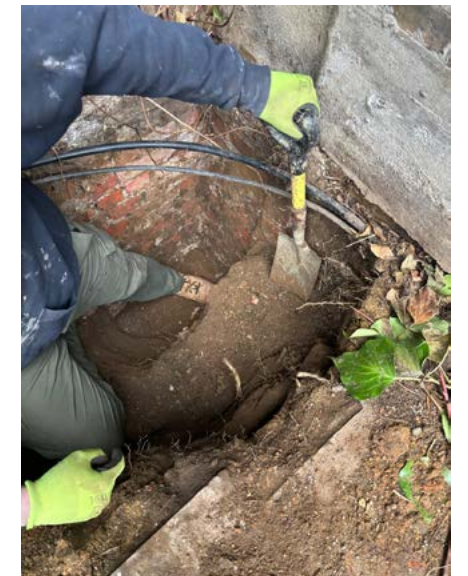
P5 - Structural investigations in the rear garden
