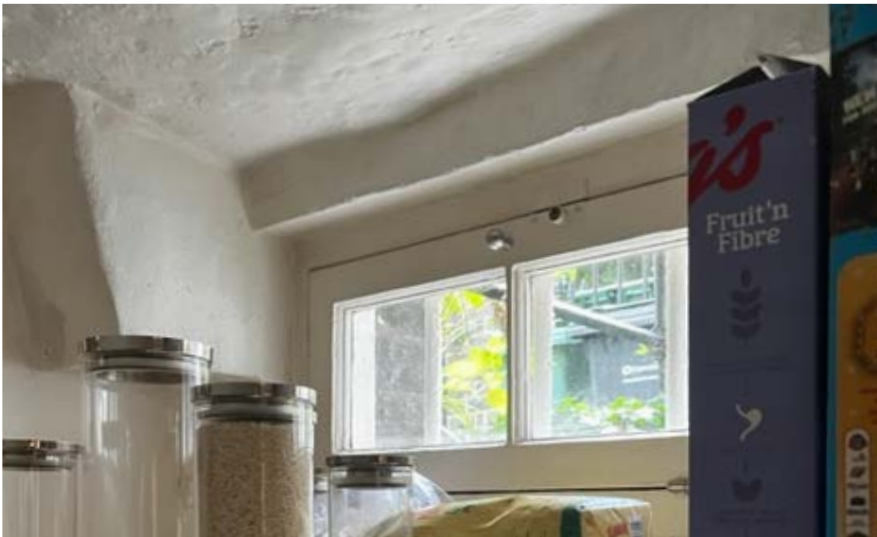
Photo from the basement. Source: Roberts & Treguer Ltd.
