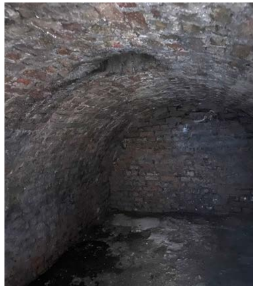
P1 - Low light photograph of coal vault with the coal hole visible at the top
