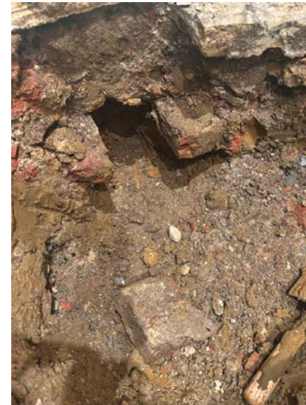
P3 - Structural investigations showing the depth of foundations in the area
