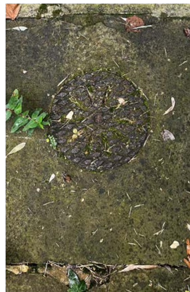
Coal hole in front of 32 Well Walk Source: R&T
