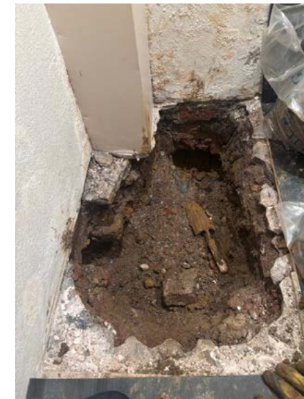
P4 - Structural investigations in the area
