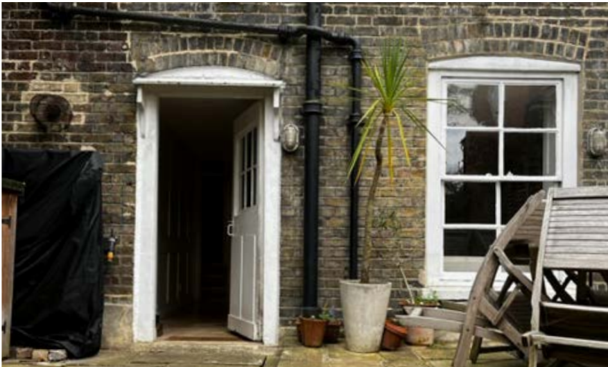
View of Rear Elevation. Source: Roberts & Treguer Ltd.
