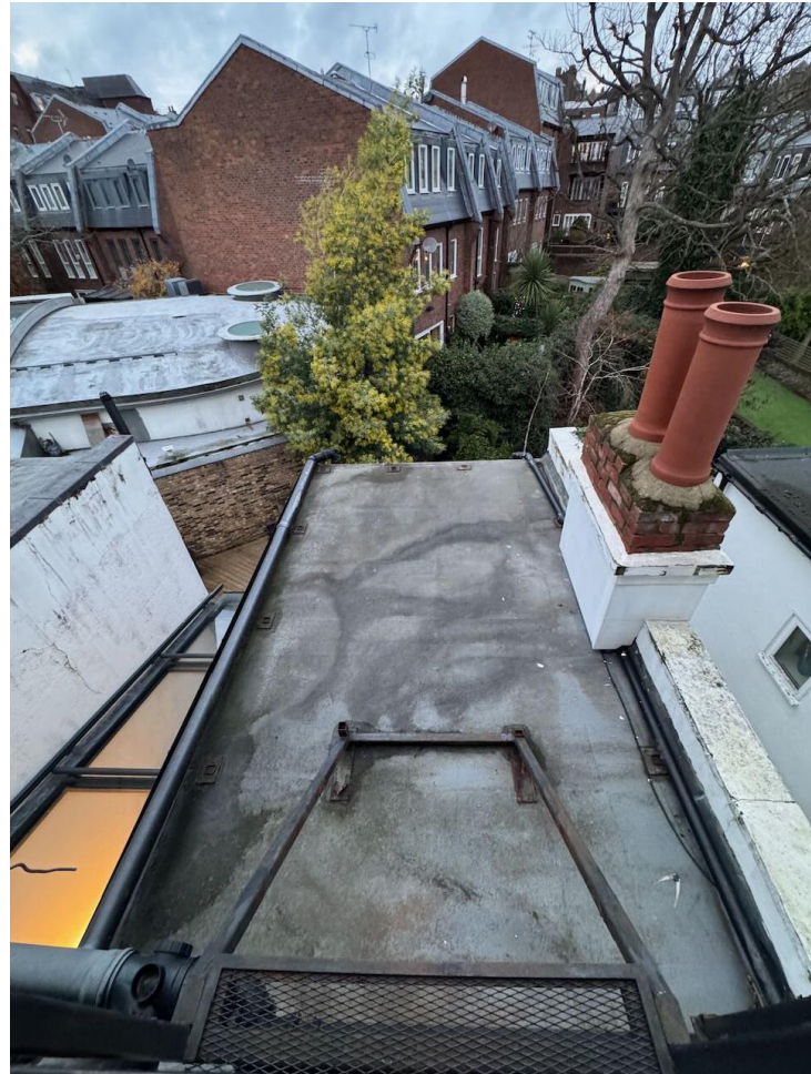
current view of outrigger roof from rear facade (second floor)
