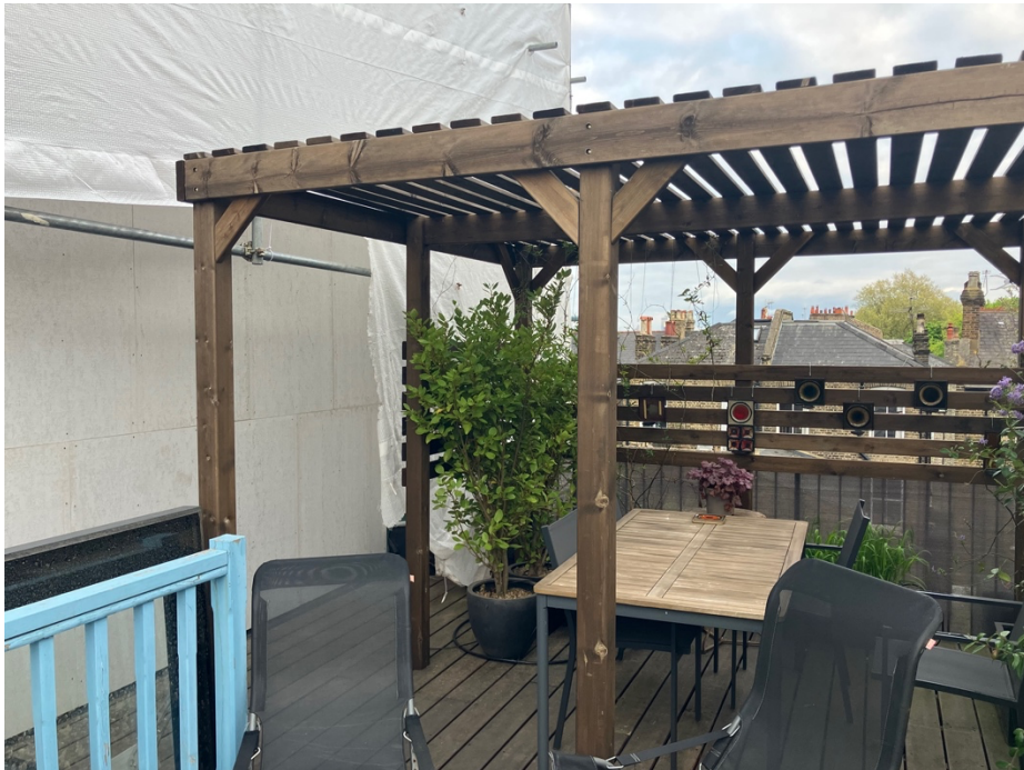
Roof terrace _ view towards the back of the property
