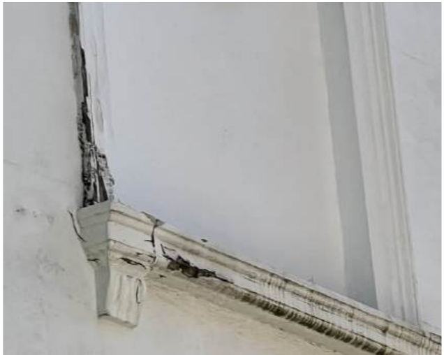
Fig.150 Deterioration of existing stucco work
