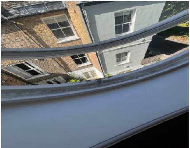
Fig.152 Deterioration of existing window frames
